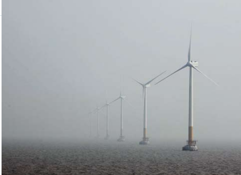
A view of East Sea Bridge Wind Farm in heavy fog
